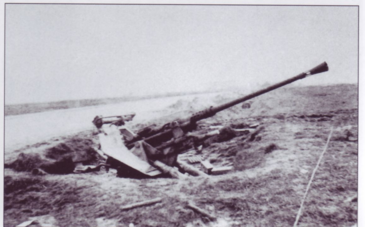
This 3.7cm FlaK36 is possibly a derelict, since very little in the way of crew gear or accessories are visible in the photograph, including any ready ammunition. Note the configuration of the gun tube with the perforations on the collar where it joins the receiver group, as well as the slots on the muzzle flash suppressor. This gun also has a partial shield on the gunner's side.
