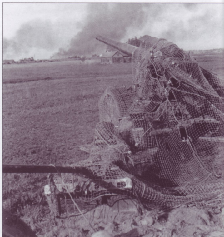
The crew of this 10cm K18 has spread netting over their gun to help conceal it a bit more on the open terrain of the Ostfront. Note that the earth spade has been properly dug in and there is large hand-spade protruding from the trail leg. The latter item was used to re-position the piece.
