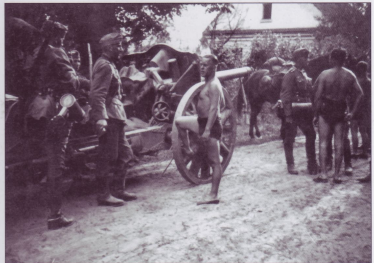
Taking advantage of the weather conditions, a pair of German troops greets their comrades wearing nothing but athletic shorts. The 10.5cm I.FH18 is still in travel mode (note the piece's attitude and the folded-up earth spades on the trail legs) and remains attached to its limber, which is off-camera.
