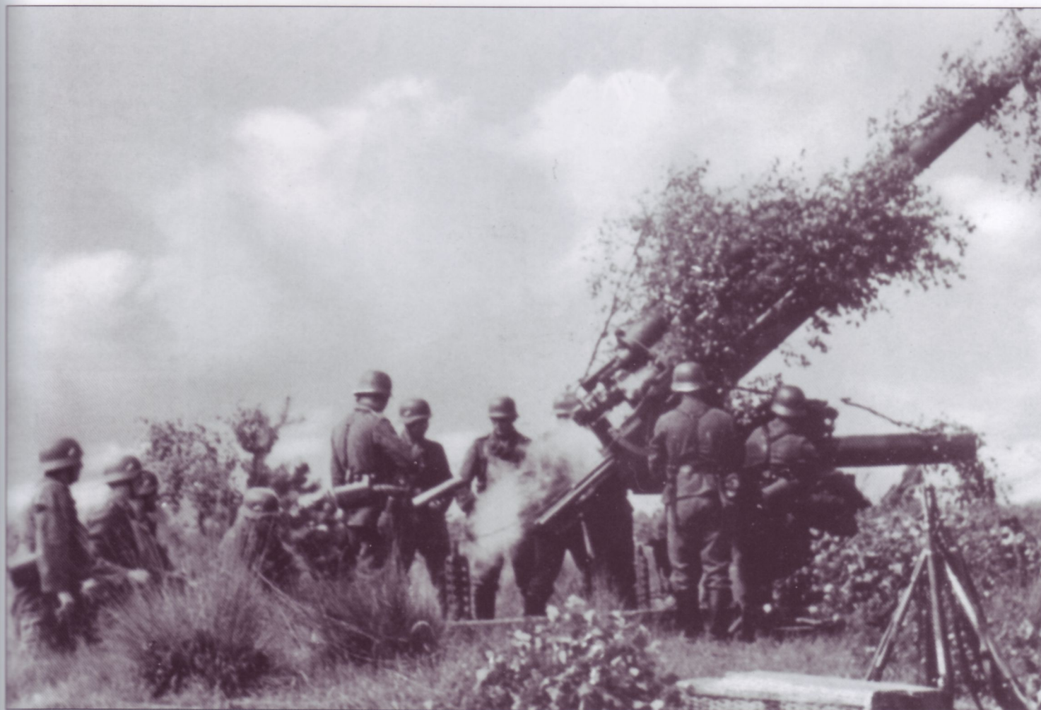
The crew of this partially-camouflaged 8.8cm FlaK18 engages an aerial target; the angle of the gun tube, the position and attitude of the gun-layer on the near side of the piece and the ammunition handlers at the ready all suggest that they are laying down an anti-aircraft barrage. The location of the earth anchor on the Kreuzlafette 18, seen just below the gas escaping from the gun breech, identifies the model type. Note also that the crew has "stacked arms" (their Kar98k rifles are hooked together in a pyramid shape) and that there is a wicker three-round ammunition container in the foreground.
