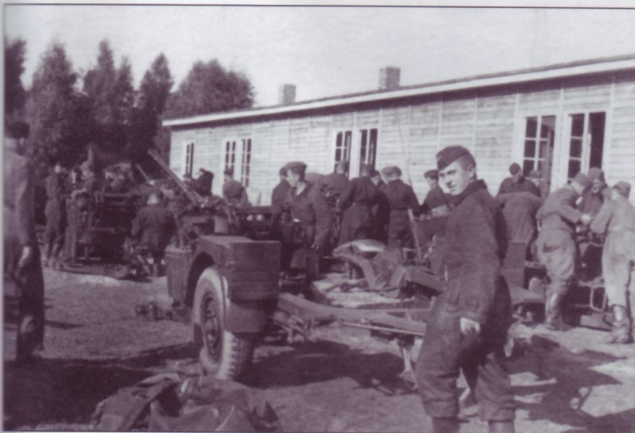
In this possibly pre-war photo, several crews work on maintaining their 3.7cm FlaK36s, in an area adjacent to their barracks. The guns have been detached from their Sd.Ah.52 limbers, affording a fine view of some details of the latter. Note also, the attitude of the limber when resting on its skid.
