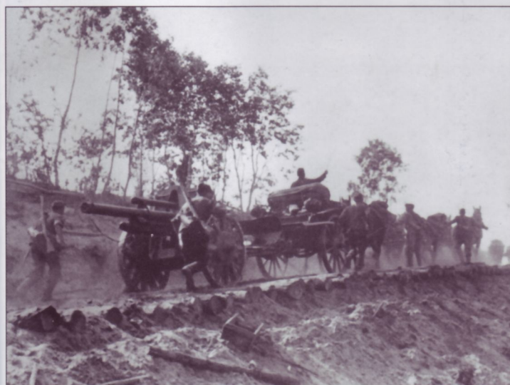
The use of so-called "corduroy" roads made from logs, as seen here, helps heavy equipment such as this horse-drawn 10.5cm I.FH18 negotiate soft ground. Note that on this incline, only the teamster is riding; the remainder of the crew, including the three men who normally rode the left-hand horses, are all on the ground, struggling to get their howitzer to its next destination.
