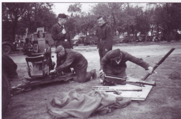
In what is also probably a pre-war training scene, the crew of this 2cm FlaK30 has partially disassembled their gun for maintenance. Note the man at right working on the receiver group, while to the left another crewman works on the platform mount. In the background are several motor vehicles, including a Krupp L2H143 (Kfz.69) tractor at left, and a number of Opel Blitz 3-ton trucks at right.
