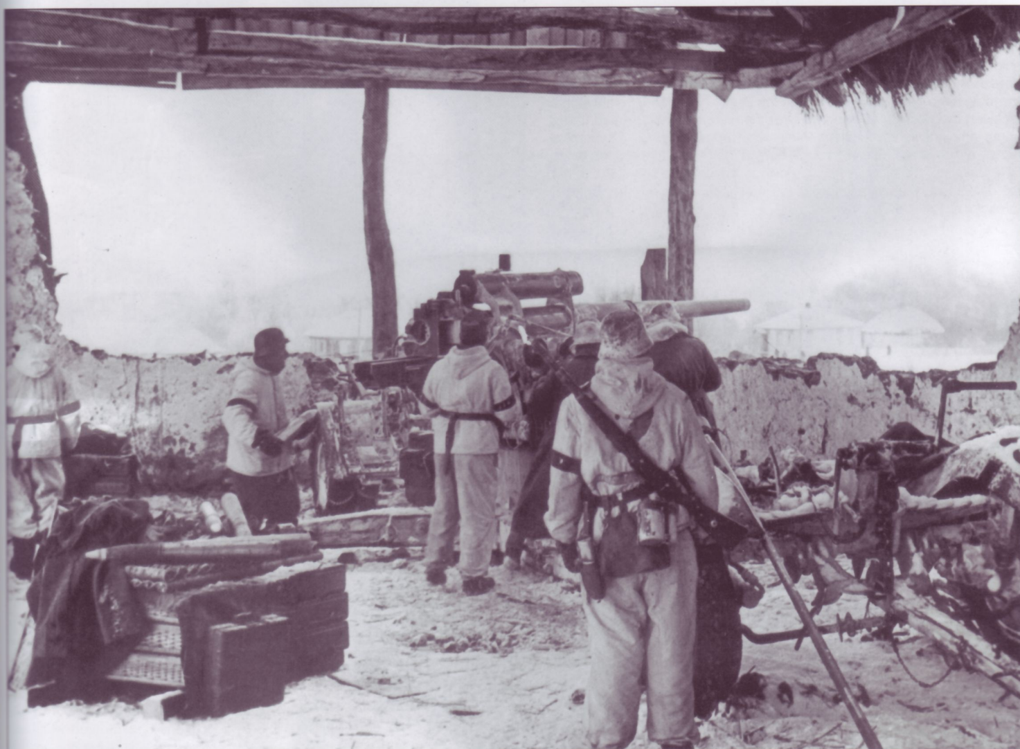
The crew of this 8.8cm FlaK18 (note the Sd.Ah.201 limber section at right) has emplaced their piece inside a partially destroyed structure. Note how the wall has been opened to provide a field of fire and the upright logs that support the roof. The crew seems to be engaging a ground target as can be determined by the elevation of the mono-block gun tube and the position of the loader, who waits with a fresh round. Note also the stack of wicker three-round ammunition containers with ready rounds on top.
