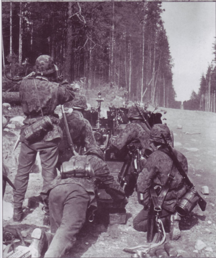
While their commander gazes through his binoculars for a target, the crew of this 7.5cm I.G.18 prepares for the order to fire. Note the man in the foreground with the unenviable task of steadying the piece since in their haste the crew has not had time to emplace the earth spade at the rear end of the box trails. Their uniforms also identify these men as members of the Waffen-SS.
