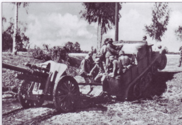
Hauled by its leichter Zugkraftwagen 3-ton Sd.Kfz.11 tractor, this 10.5cm I.FH18 is just about to negotiate a ditch on its way to the front. It appears that some retouching was carried out on the original photograph; note the wheels on both the howitzer and the tractor.
