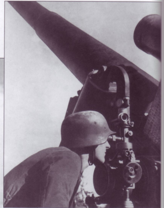
A helmeted gun-layer peers through the sight of his 21cm Mrs18. This close-up provides some details of the various parts of the sight, as well as showing the range-data table at right.
