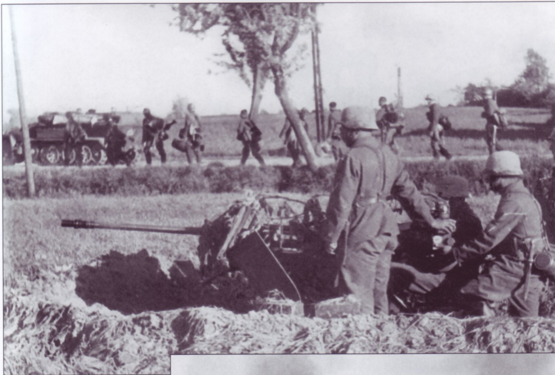
An emplaced 2cm FlaK30 covers a road as infantrymen and an Sd.Kfz.251 Ausf.A or B advances. This gun also has a splinter shield fitted and it seems that the crew have used mud to tone down their helmets for concealment.
