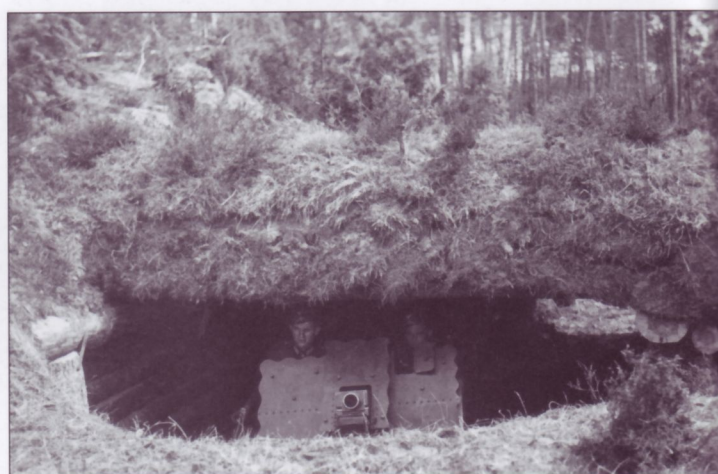
When the situation allowed for it, German troops would often "make themselves at home" by constructing rather elaborate field works as seen here. Two crew-members assigned to this 7.5cm I.G.18 peer out from their earth and log bunker. They have carefully covered the position with sod, which will help better conceal them from the prying eyes of the enemy.
