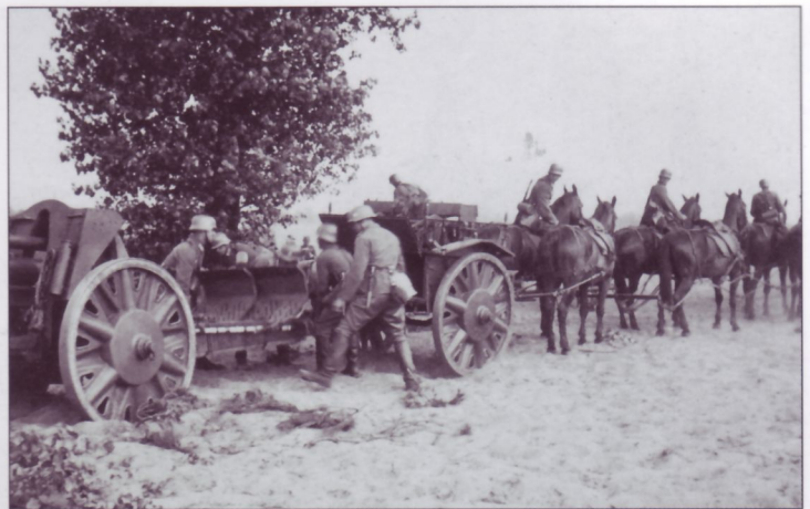
The majority of the guns fielded by Germany were designed also to be drawn by horses, as seen here. This 10.5cm I.FH18 is attached to a limber, with the whole being moved by six horses; note the wheel configuration of both the howitzer and the limber. Note also the relatively large size of the earth spades at the tips of the trail legs, which are folded up and forwards for travel.
